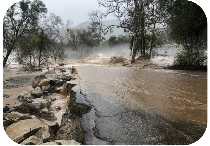
North Fork Drive and Bridge covered in rushing water from the North Fork of the Kaweah River. Image Credit: Julia Goolsby.
